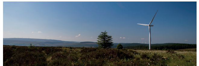
Castle Craig Wind Farm, Northern Ireland (turbines 125m to blade tip) ©KeithArkins
